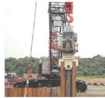
Photo 5 Condition of vibratory driving
