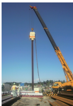
Photo 13 Condition of application for temporary retaining wall
