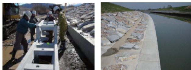
Photo 8 Precast concrete cooping of hat-shaped steel sheet pile 3)
