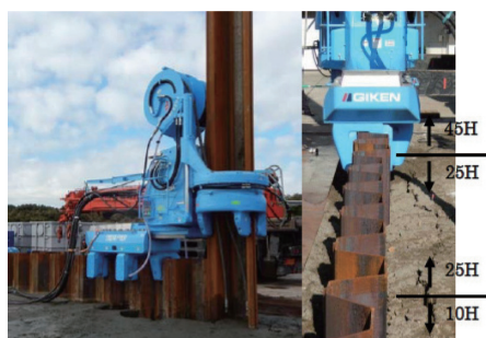
Photo 6 Condition of hydraulic jacking driving
