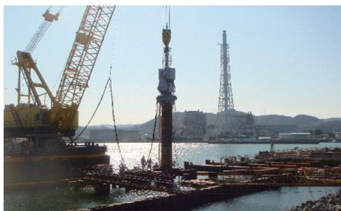
Photo 5 Construction of RS Plus™ method on the Karatsu Port
