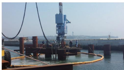
Photo 7 Construction of RS Plus™ method on the Onahama Port
