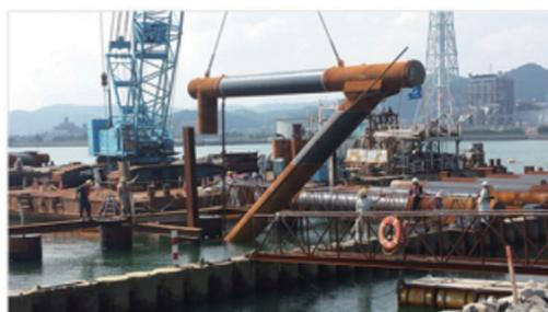
Photo 6 Installation of submerged strut members on the Karatsu Port
