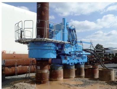
Photo 6 Driving test by Gyropress method
