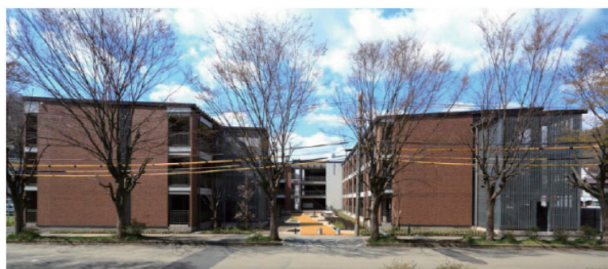
Photo 12 3-story restoration public housing in Kamaishi, Iwate (NS-SUPER-FRAME™)
