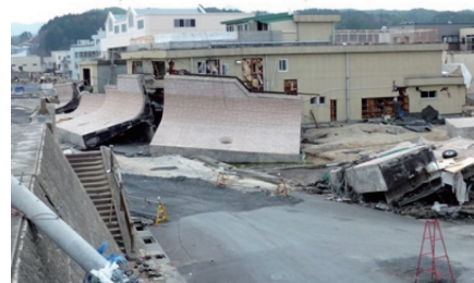
Photo 3 Devastated breakwaters and tide barrier
