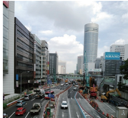
Photo 6 Construction of steel diaphragm wall with soil cement
