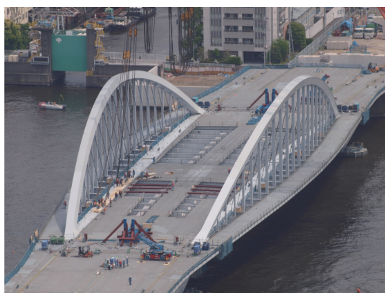
Fig. 4 Tsukiji-ohashi Bridge applied over 50 mm thickness SBHS500 around panel point sections
