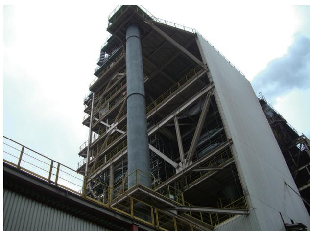
Fig. 14 Coal perpendicular conveyor duct of ARU-TEN
