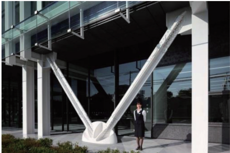
Fig. 7 Appearance of energy dissipative brace and column applied BT-HT880
