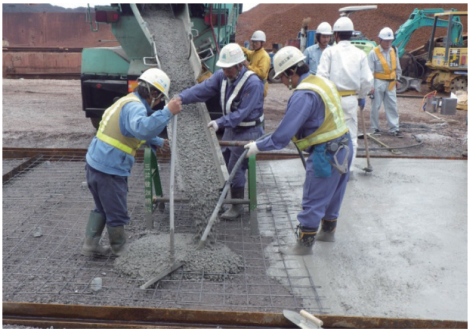
Photo 5.1 Placing of concrete
