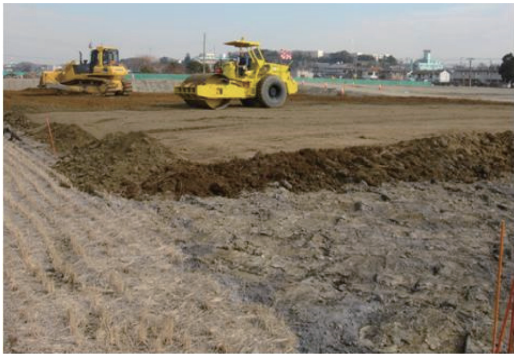
Fig. 3.5 Construction situation of the soft ground improvement
