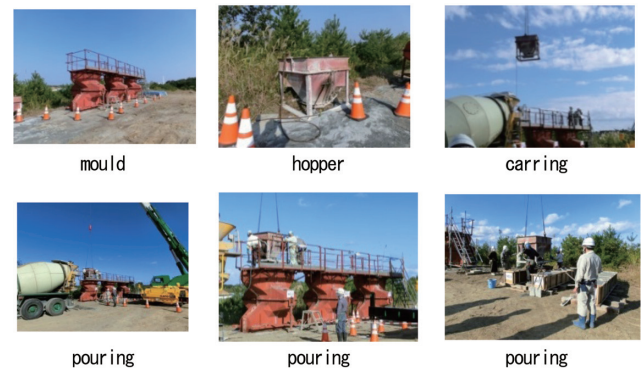
Photo 1.4 Concrete placing situation
