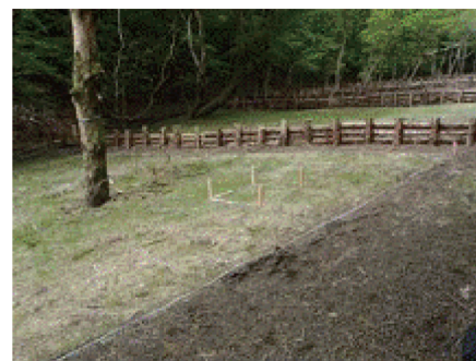
Photo 8(c) After construction
