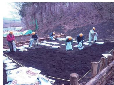
Photo 8(b) Under construction
