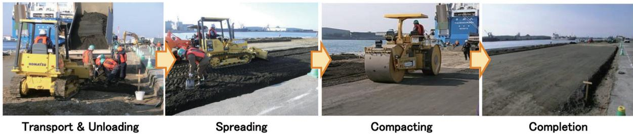
Photo 2 Example of construction (Sendai Shiogama Port)
