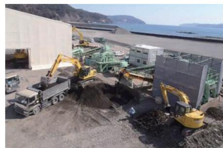
**Photo 1 High-speed rotary CaO-improvement plant (disaster waste recovery project of Kamaishi City, Iwate)**
