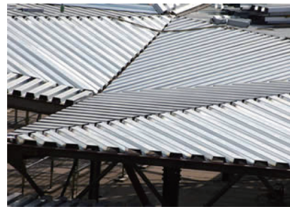
Fig. 11 Corrugated sheet roof
