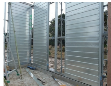
Fig. 12 Corrugated sheet wall
