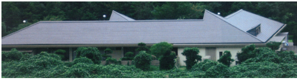
Fig. 8 Example of chromate-free prepainted steel applied to roof materials (February 2009)
