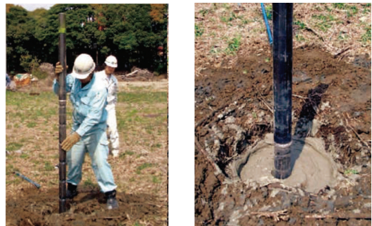
Fig. 4 Example of ground improvement work using grooved pipes
