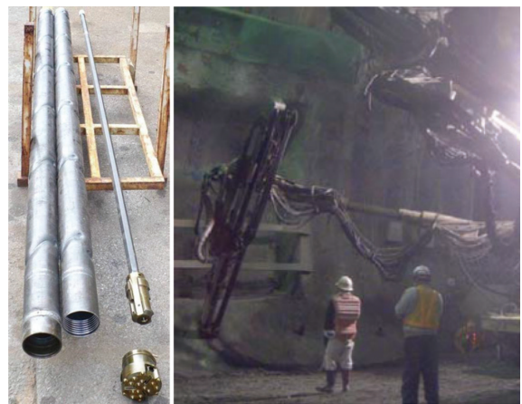
Fig. 5 Oblique-grooved pipes (left), and foot piling work for tunnel 5)
