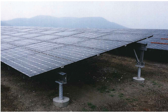
Fig. 14 Application Example: Pilings for solar panels
