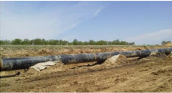
Fig. 18 Field construction line of API X60 high-deformability linepipes<sup>6)</sup>
