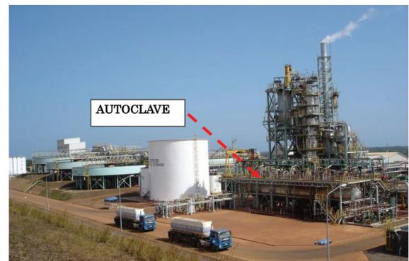
Photo 3 Nickel refining plant which applied corrosion-resistant titanium alloy for its autoclaves
