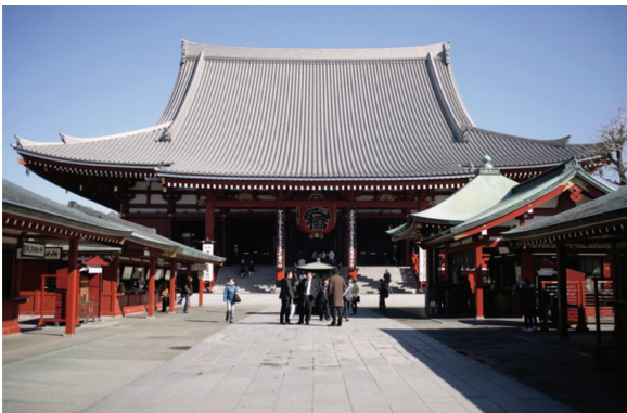
Photo 6 Titanium roof of Sensoji Temple Main Hall
