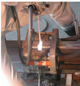
Photo 7 Example of continuous welding process in the enclosed-arc welding
