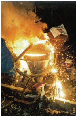
Photo 5 Example of thermite reaction process
