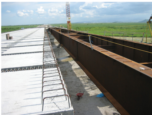
Photo 1 Two main steel girders on Subic-Clark Tarlac expressway construction in Philippines
