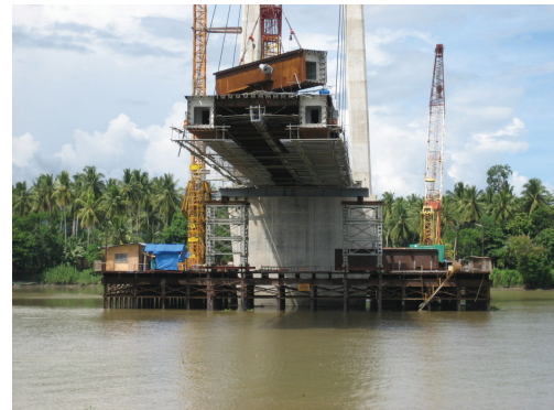
Photo 5 Steel box girder construction of Second Magsaysay Bridge
