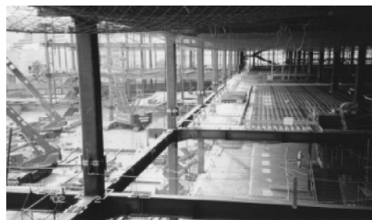
Photo 3 Building erection using SHTB
