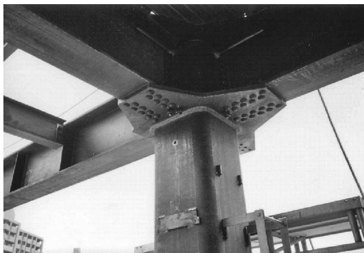
Photo 5 Beam-column joint using SHTB
