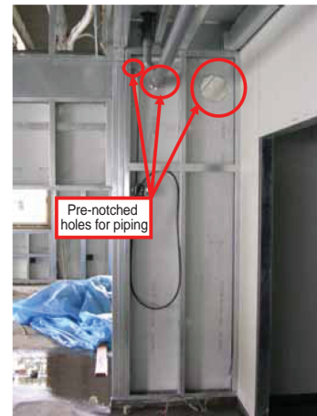
Photo 17 Pre-notched holes for piping penetration to structural face board
