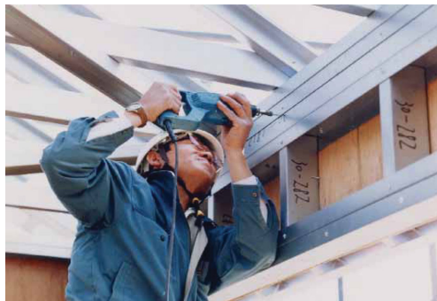
Photo 2 Scene of joining with drilling tapping screws
