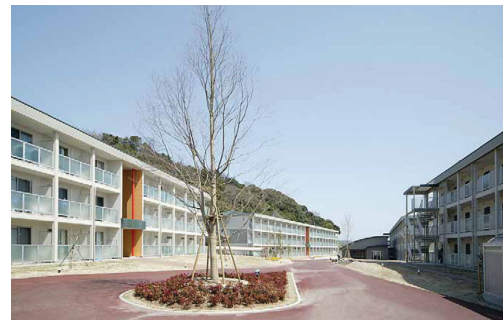
Photo 13 Three-story dormitory for foreign students in Kitakyushu City (60-minute quasi- fire-resistant building)
