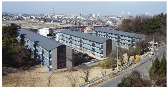
Photo 14 Three-story apartment for employees of Nagoya Works in Takayokosuka, Aichi (1-hour fire-resistant building)
