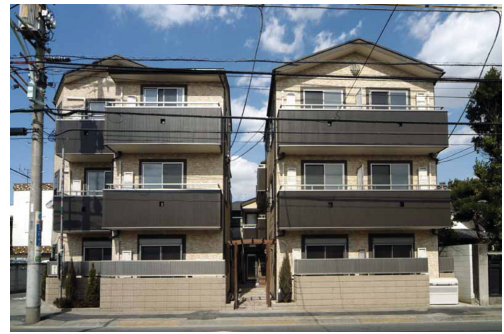
Photo 12 Three-story apartment, city type and narrow small area, in Chofu City, Tokyo (1-hour fire-resistant building)
