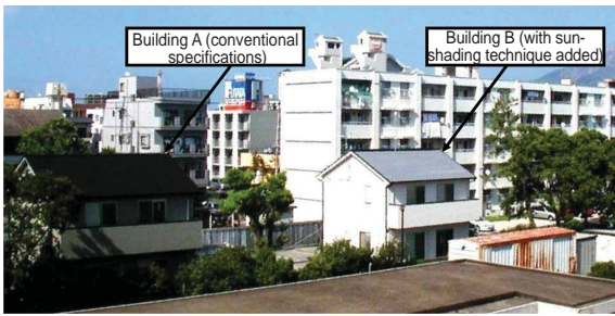
Photo 7 Two-story detached houses for on-site practical study at Kagoshima University
