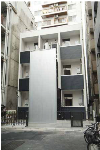
Photo 11 Three-story apartment, city type and narrow small area, in Minami-Ikebukuro, Tokyo (1-hour fire-resistant building)
