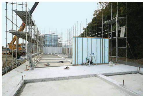
Photo 6 Exterior wall panels, increasing ratio of factory production
