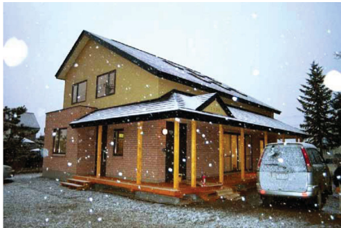
Photo 5 Steel framed house constructed in Engaru City, Hokkaido
