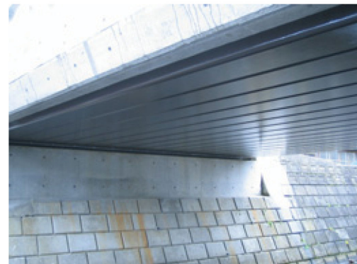
Fig. 11 Completed Kosawada bridge
