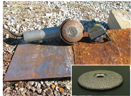
Fig. 12 Removing of thick adherent rust on weathering steel by a developed instrument
