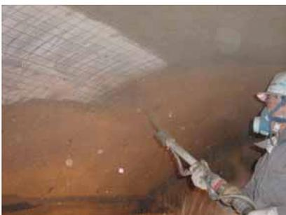
Photo 1 Spray mortal type fire refractory
