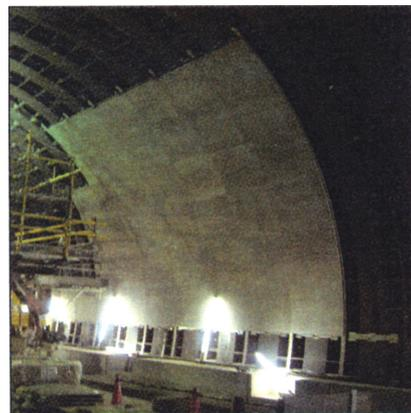
Photo 2 Board type fire refractory
