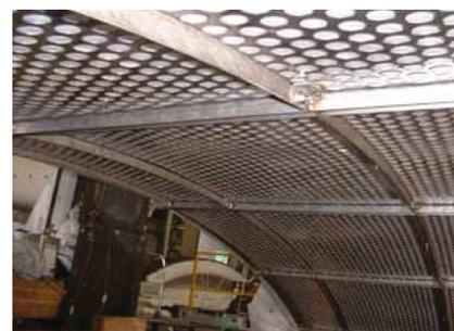
Photo 3 Fiber blanket type fire refractory with stainless steel
