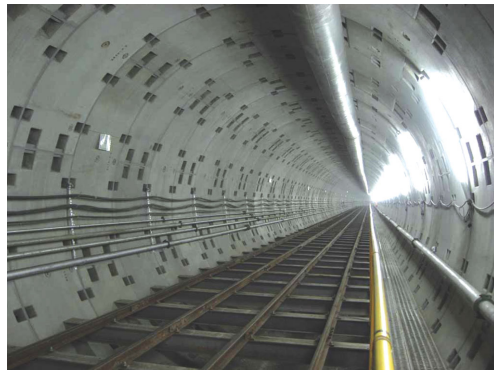
Photo 4 Shield tunnel constructed with CP segments
