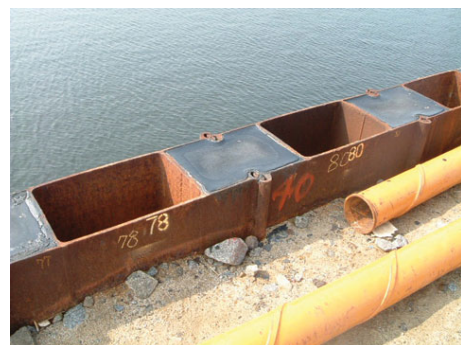
Photo 8 Steel hydraulic barriers using NS-BOX
