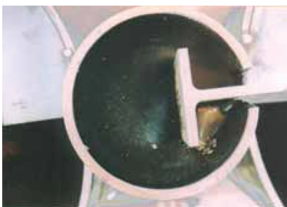
Photo 7 Steel sheet pipe pile joint filled with asphalt compound
