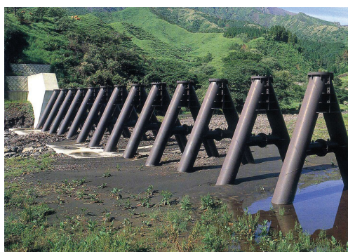
Photo 2 Slit dam A type (permeable-type steel dams)
