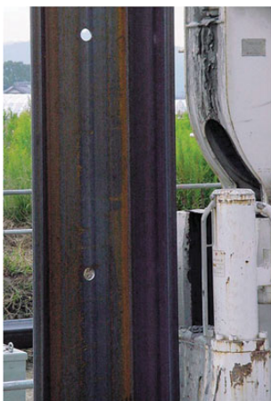
Photo 1 Water-permeable steel sheet pile
