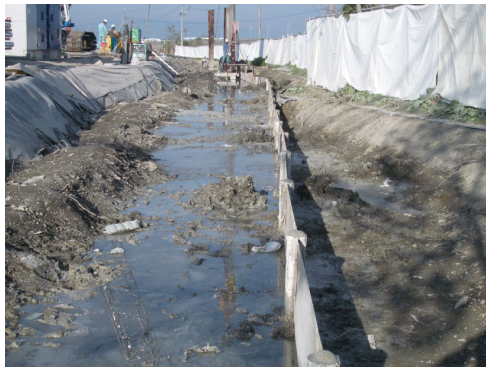
Photo 9 Steel liner sheet with water cut-off joint
