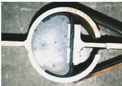
Photo 6 Steel sheet pipe pile joint with leakage prevention rubber sheet
