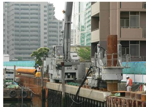
Photo 7 Gyro-press construction site example 1
