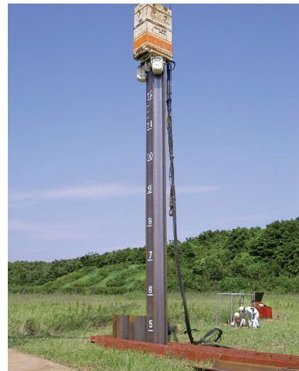
Photo 2 Driven Hat-Type Sheet Pile 900 by vibratory driving
