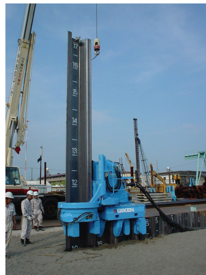
Photo 3 Driven Hat-Type Sheet Pile 900 by hydraulic jacking method
