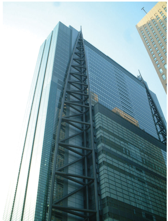
Photo 1 Nippon Television Network Corporation Tower using buckling restrained brace
