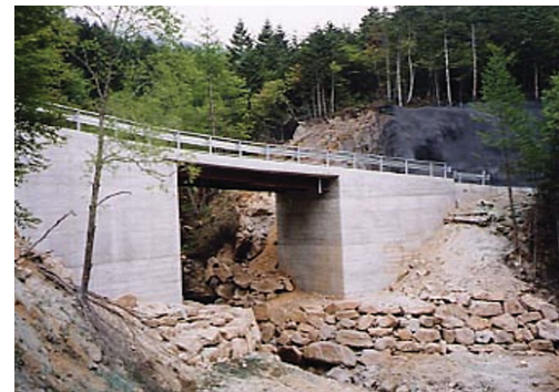
Photo 10 Construction of HBB with rigid beam ends
