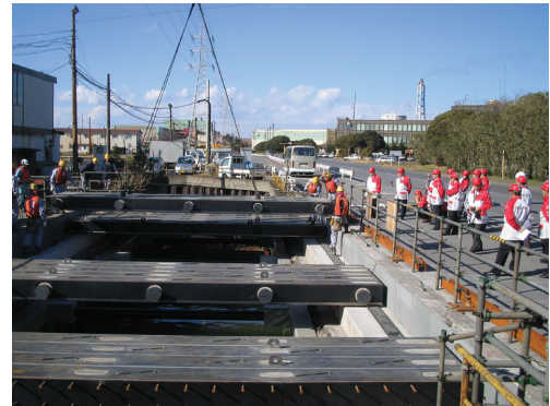
Photo 9 Construction of Kakutabashi at Kimitsu Works
