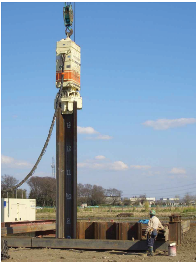
Photo 6 Hat type sheet pile driving
