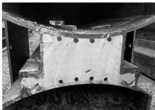
Photo 4 High Capacity and Broad type steel sheet pile junction
