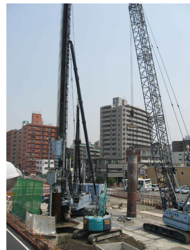
Photo 1 Gantetsu Pile construction method
