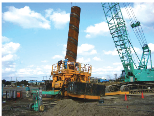
Photo 2 NS-Eco-Pile construction method
