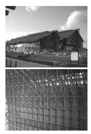
Site area: 26,485 m<sup>2</sup> Building area: 12,040 m<sup>2</sup> Floor area: 15,894 m<sup>2</sup> Structure: Timber + reinforced concrete Roof: Timber reinforced with steel Number of stories: 1 underground, 2 above ground Maximum height: 39.89 m Timber structure construction period: From July to December, 2002
