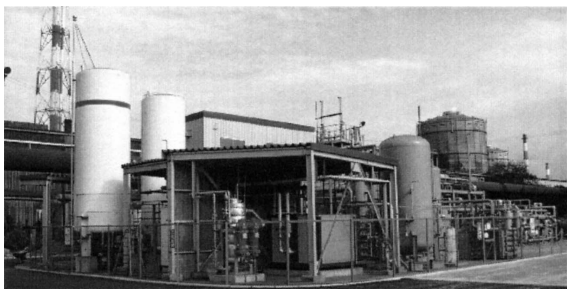
Photo 1 Cover view of the plant
