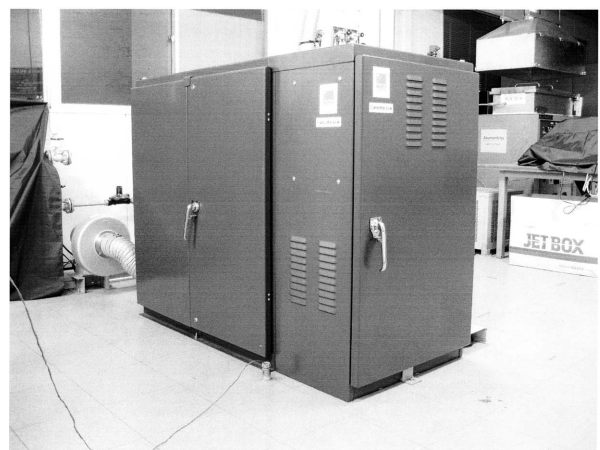
Photo 1 2kW SOFC in Yawata Works
