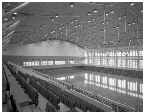
Photo 1 Tension structure No.1 (roof system)
