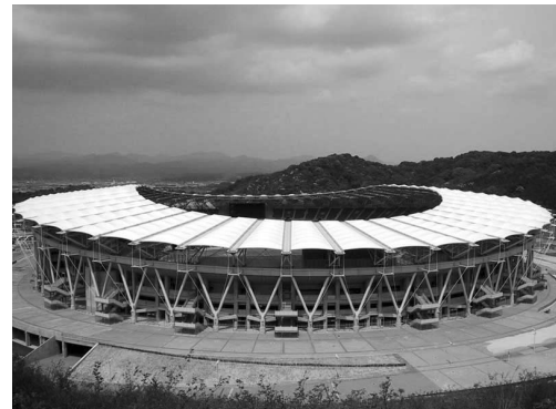
Photo 9 Constractional case (stadium)
