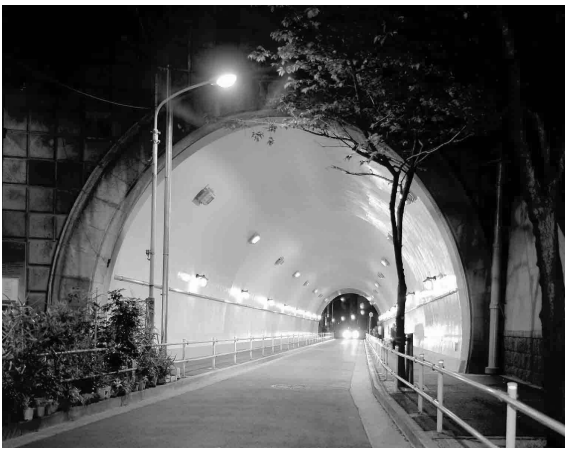
Photo 5 Example of road tunnel
