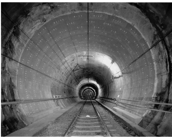
Photo 2 Example of construction for subway tunnel
