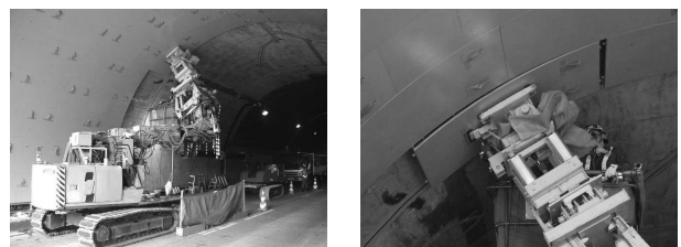
Photo 3 Installation of panel by elector machine
