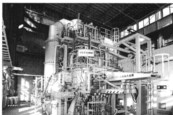
Photo 2 Overview of test plant
