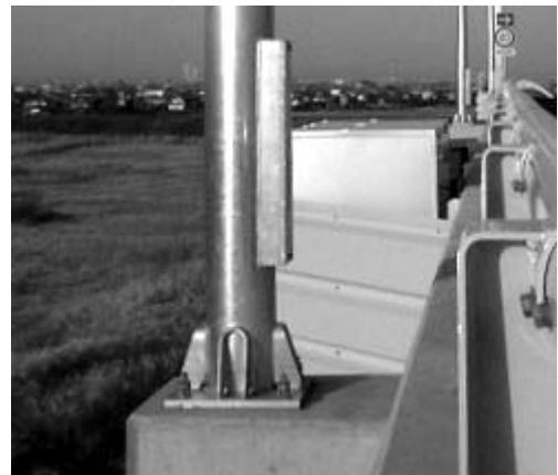
Photo 3 U-shaped rib structure
