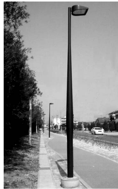
Photo 2 Entasis tapered lamp post
