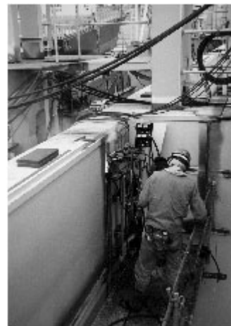
Photo 6 An example of construction site where two-electrode VEGA® operated
