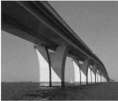
Photo 3 Piers of Tokyo TTB ( Trans-Tokyo Bay Highway) [titanium-clad steel sheet]
