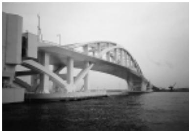
Photo 4 Pontoon of Yume - Mai Ohashi Bridge [Osaka City / titanium-clad steel sheet]
