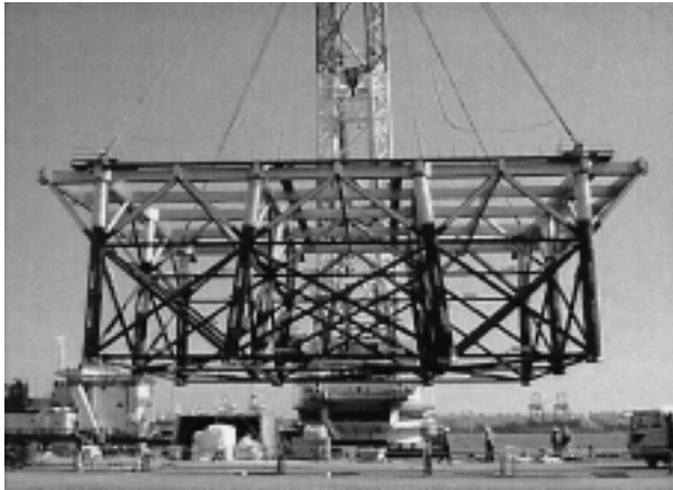
Photo 1 Example of application of seawater-resistant stainless steel sheathing (jacket type wharf)
