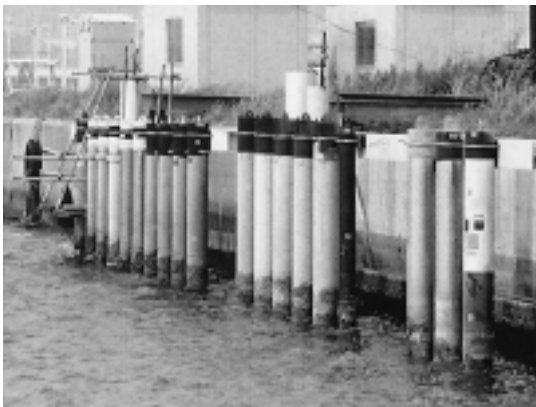
Photo 4 Marine exposure test of steel pipes with YUS270 sheathing
