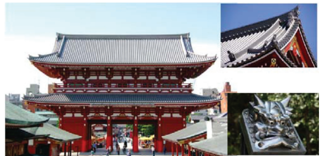
Fig. 2 Hozomon gate with titanium roofs at the Sensoji temple Upper right: Close look at the corner of the roof, Lower right: Ridge-end tile "Onigawara" made of titanium
