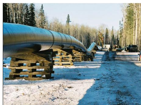
**Fig. 3** View of field construction of X120 line pipe
