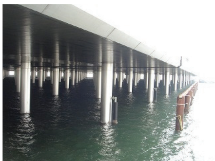
Fig. 10 Stainless steel cladding protection (Haneda Airport D-runway)
