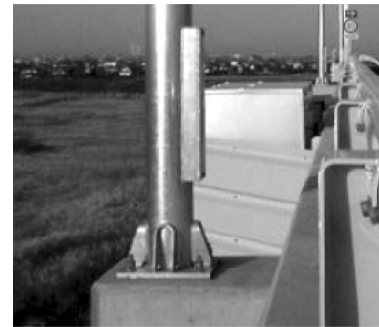
Fig. 9 U-shaped rib stiffening pole
