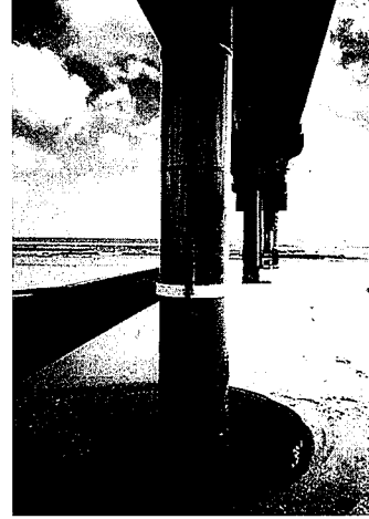
Photo 10 Research pier for field measurement in the nearshore Hasaki (1999)
