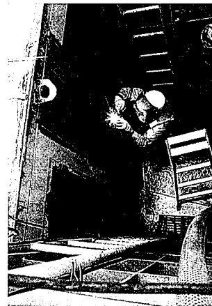
Photo 3 Applying the lining in the chamber
