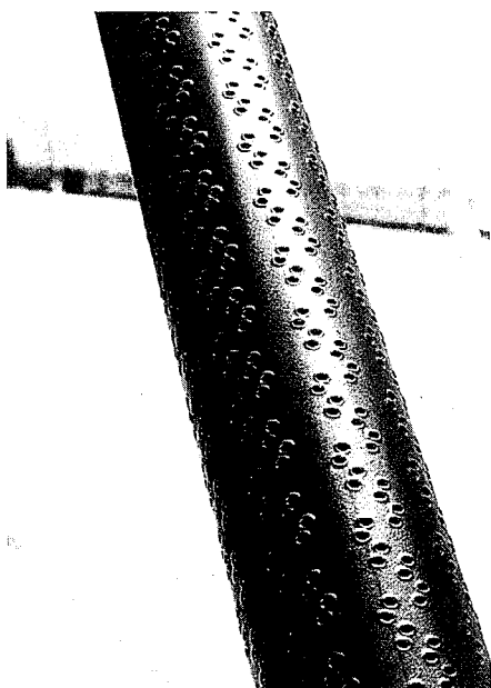
Photo 2 Indented cable of the Tataru Bridge
