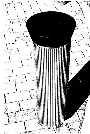
Photo 3 Trapezoidal-fluted steel pipe used in street fixtures
