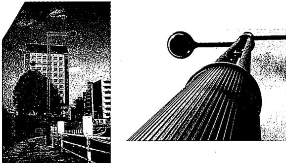
Photo 2 Trapezoidal-fluted steel pipe used in lower part of lighting pole
