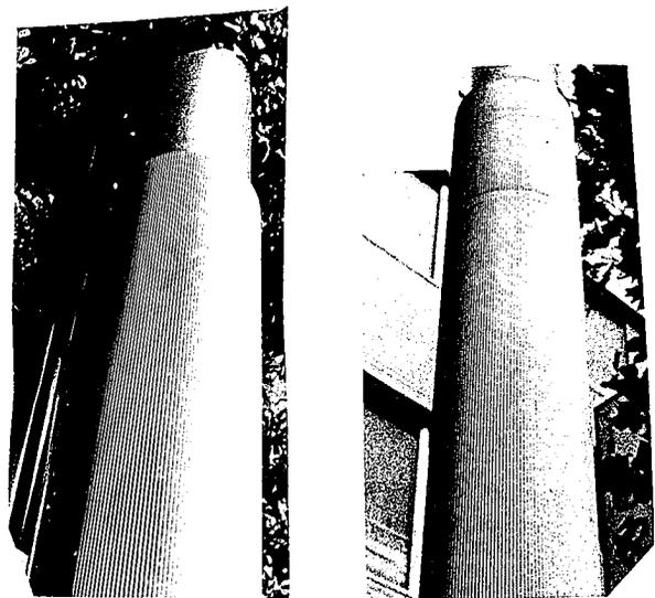
Photo 4 Sinusoidal-fluted steel pipe used as signpost
