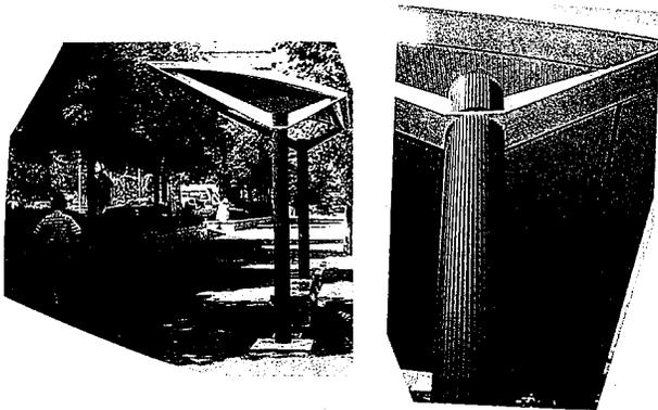
Photo 1 Trapezoidal-fluted steel pipes used as shelter columns
