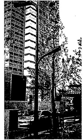
Photo 6 Taper steel pipe used as lighting pole
