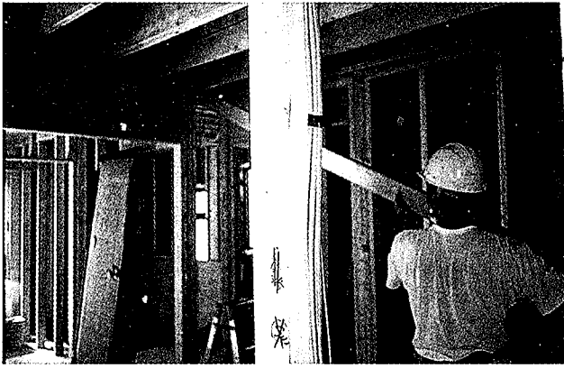
Photo 4 Operation scene of steel hanging system
