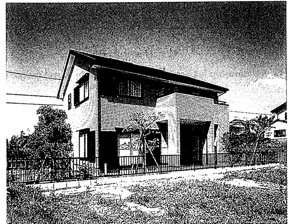
Photo 1 Steel-framed house subjected to vibration test (owned by Japan Development Co.)
