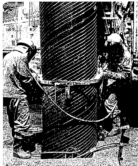
Photo 4 Site welding of steel pipe with outside surface projections
