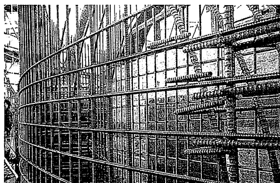
Photo 6 Placement and assembly of CFRP rods as concrete reinforcement for NOMST method
